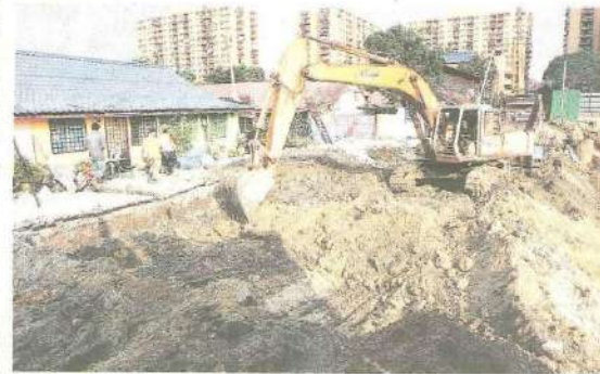
Work to clear the site of the cave-in has started.
