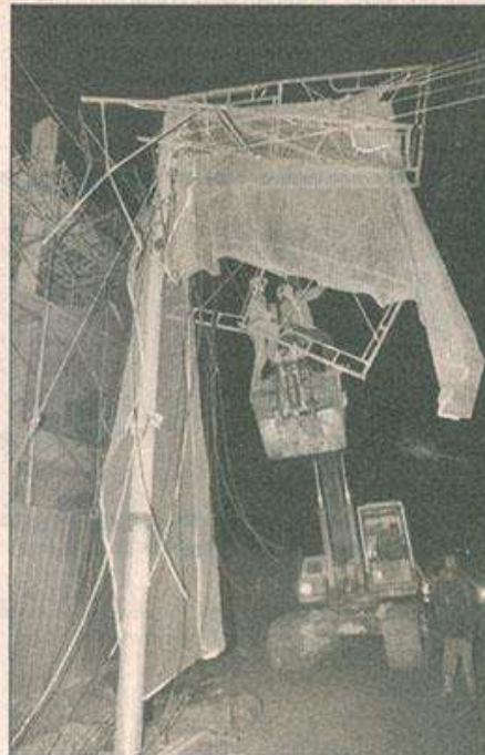
RIGHT: Work to dismantle the collapsed structure carried on at night
