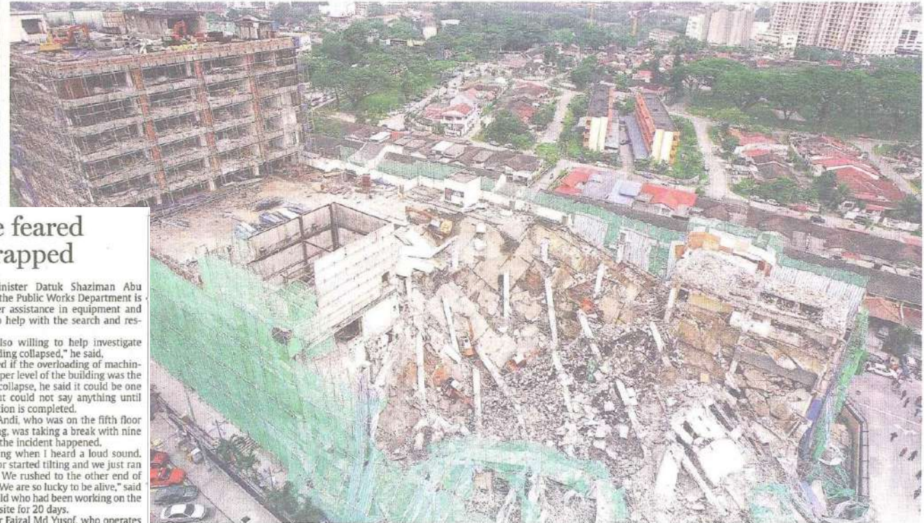
Once an icon: The old Jaya Supermarket building that was once a landmark in Petaling Jaya is now reduced to a rubble after it collapsed at about 5pm yesterday.
