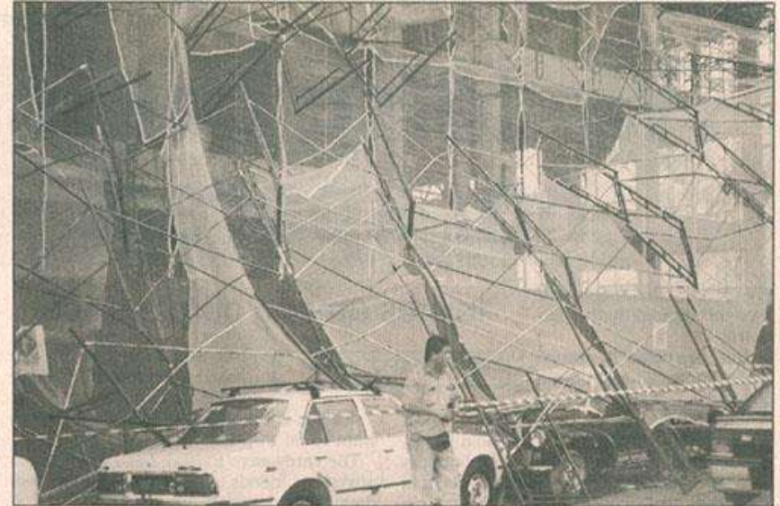
ABOVE: The fallen structure in Puchong
