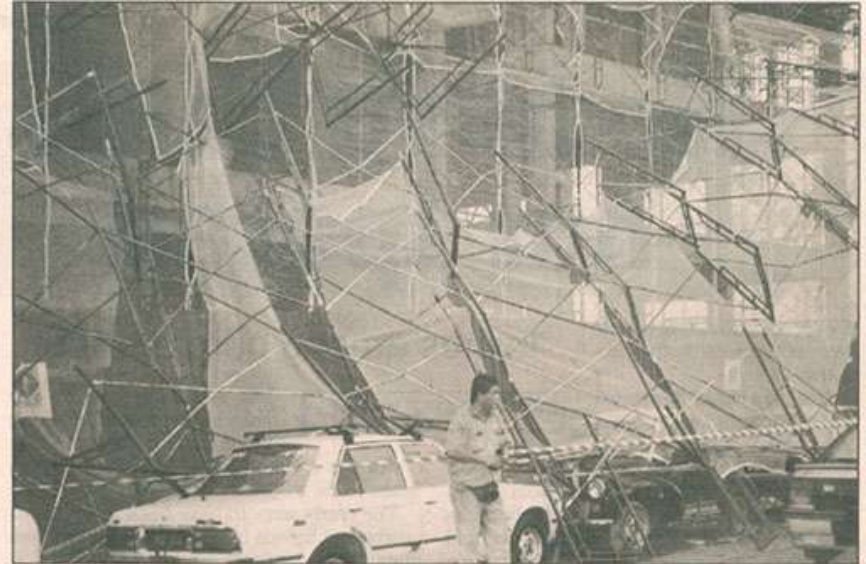
ABOVE: The fallen structure in Puchong
