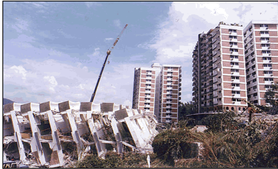
Highland Tower Collapse, 1993
